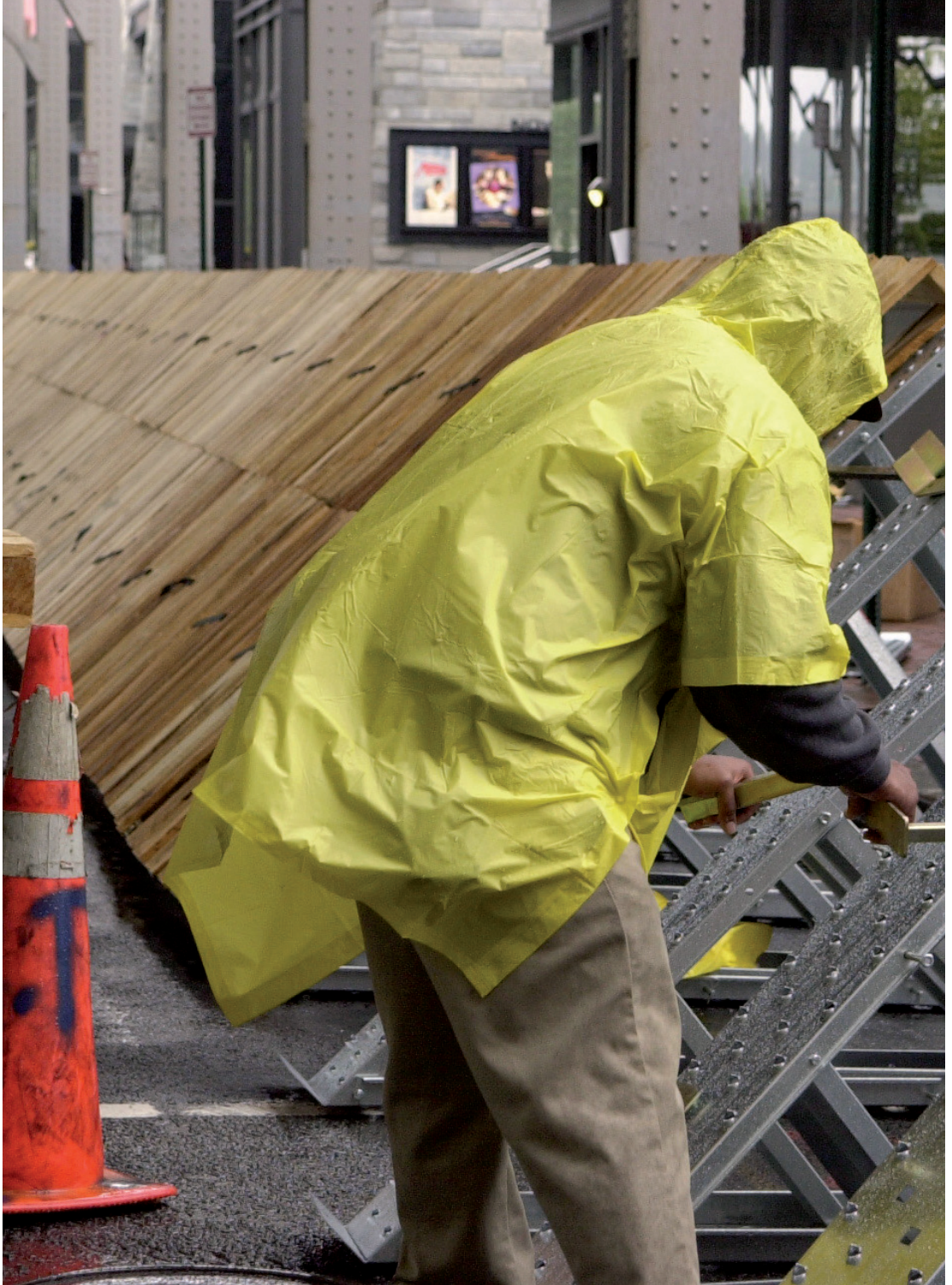
Workers construct a flood wall to protect buildings in the United States. Source: FEMA/Liz Roll.
