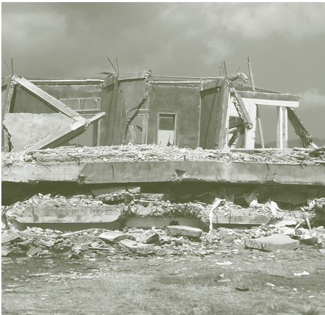
The earthquake that caused the tsunamis of 26 December, 2004 destroyed this building in Banda Aceh. This is an example of a 'soft storey' building failure that simple earthquake-resistant construction measures can prevent (for an extra 5% of the building cost).
