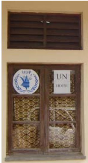
Figure 5: Shared working space in Caia
